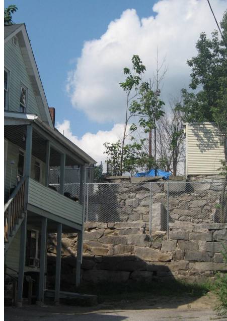
Site where a condemned barn stood at 7 ½ Ridge Street will become new Habitat home.
